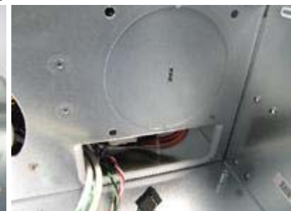
80mm fanpreparation on top of the protected cable hole
